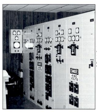
The Point Eight Power control panel for both EMD 16-645-Ideal generator sets which provide 100% backup power for the electric motor driven pumps.
